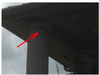
Maintenance Repair Fascia: Wood - Paint is worn / peeling Maintenance Repair Soffits: Wood - Damaged paint finish, Damaged, Siding damage at front columns from bird damage
