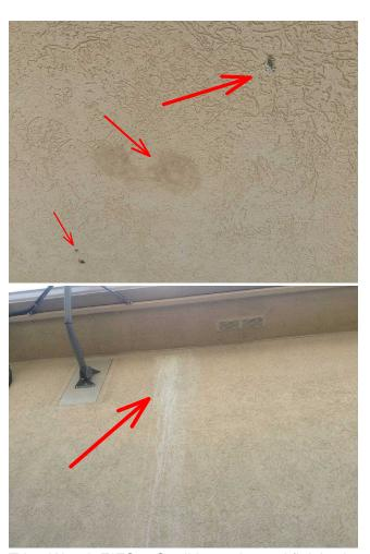
Maintenance Repair Trim: Wood, EIFS - Caulking paint and finished needed, Evidence of prior repairs to the south side of the residence building
